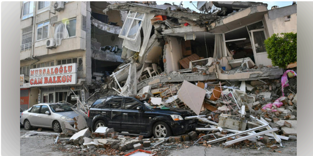
📌 A magnitude 5.4 earthquake just struck eastern Turkey with severe shaking — the ground lurched hard enough to crack walls near the town of Sincik © oskaycaglar/Unsplash
